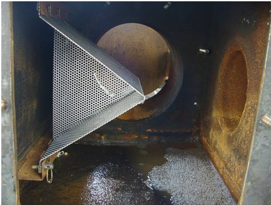
Figure 2. Client's Flameout FTPS Type B Foam Maker and Foam Chamber (Rear View).
